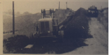
This scene will be repeated many times in all areas of the lake until mains are completed to serve all lot owners.
