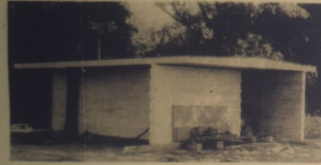
This is the new pump house and supply tank shelter, completed recently by the water department, awaiting power around service.
